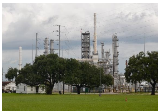
Top: Valero facility fencing displaying community banner. Bottom: Community park and housing adjacent to Valero facility in the background. (OIG photos)
