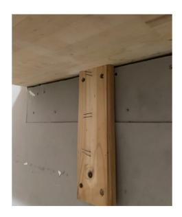
Not only was the counter unsupported and not attached properly (and therefore lifting off), but the wall it was on was not finished and had bare drywall with exposed seams. The bracket that was installed was not attached properly and broke off, leaving it in a dangerous state with exposed nails that the tenants' children could easily injure themselves on.
