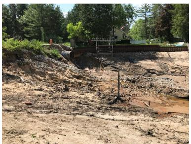
Photo from 6/10/20 culvert under E Lakeshore Dr. on Wixom Lake showing lowered water levels in Wixom Lake; 1) tall unvegetated banks of fine grained (sand and silt/organics), unconsolidated material actively eroding into the stream channel; 2) culvert shown perched above dry lake bottom – fish cannot swim from below the culvert to the stream channel above the culvert due to the difference in water levels.
