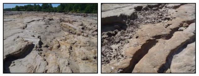
Figure 4 Reservoir bed scouring.
