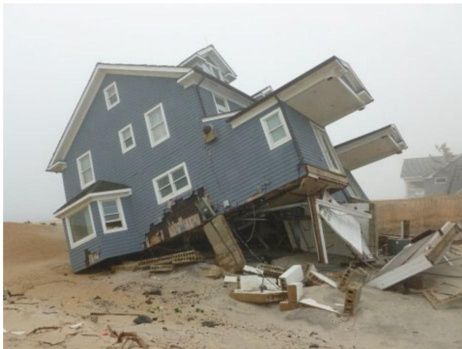
**Figure 13: House in Mantoloking Knocked Off Foundation by Superstorm Sandy Storm Surge<sup>284</sup>**
