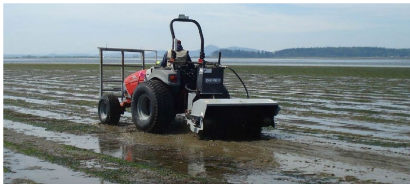
21 Figure 6: Tractor with Street Sweeper, Willapa Bay
